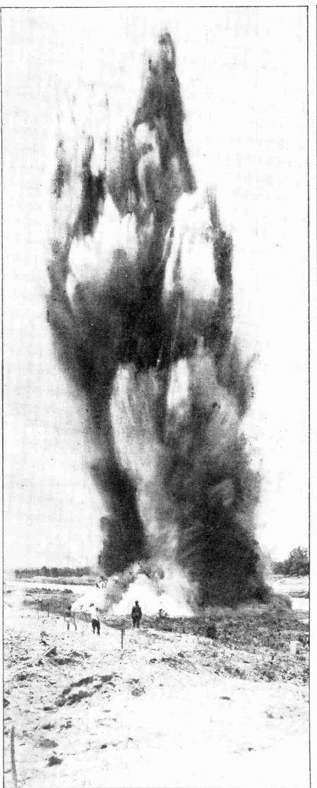
One of the most interesting jobs ever done by dynamite has been the use of it in many parts of the country to make new courses for streams. Above is a dynamite blast which built a new channel for a stream in Mississippi
