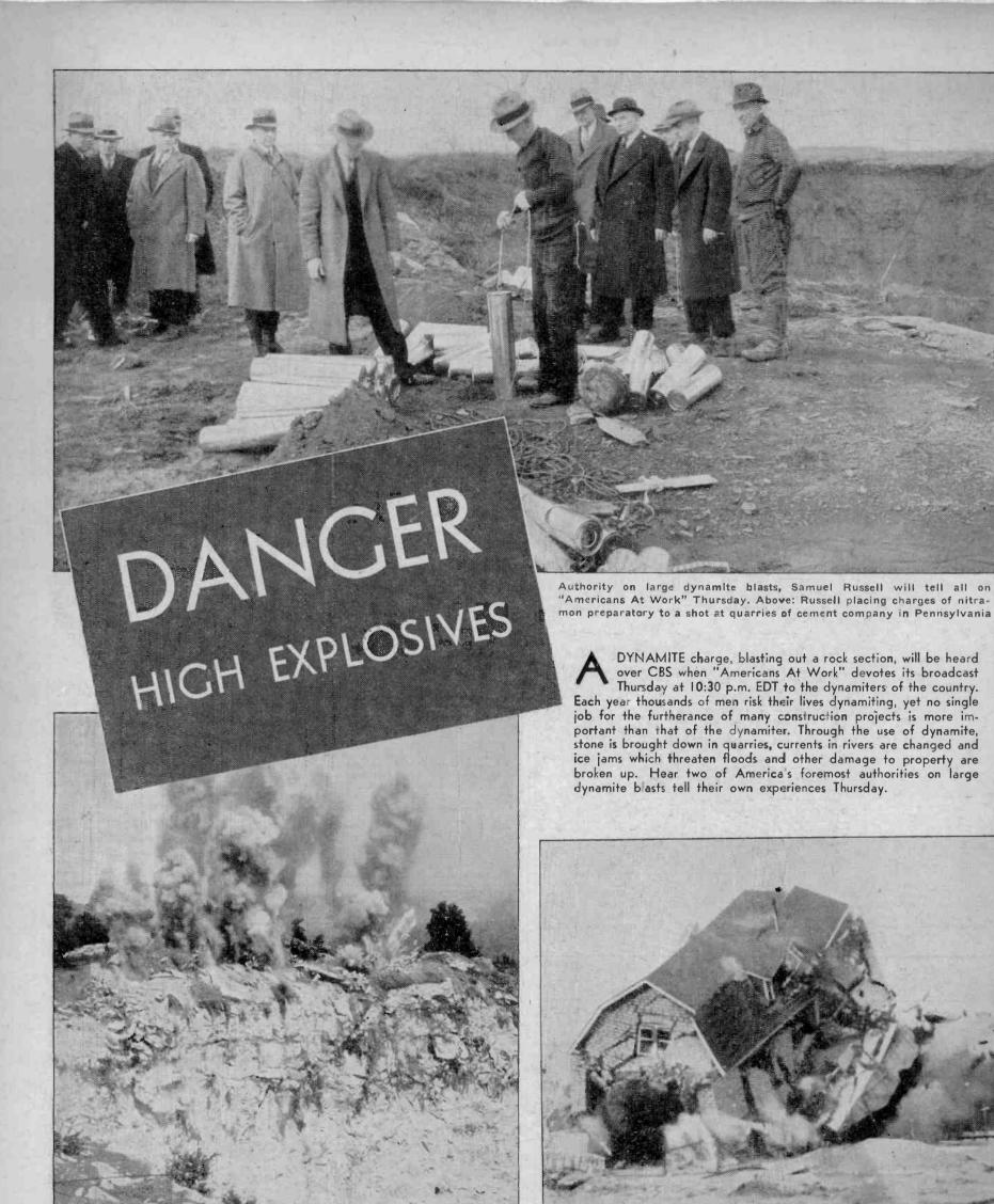
In some quarries dynamite shots are used to bring down the stone. Tunnels are driven into the side of a hill and dynamite is placed in the tunnels. This picture shows such a tunnel-shot as dynamite explodes
